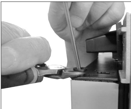
7. Remove the bush and door closer by use of a pincher.
